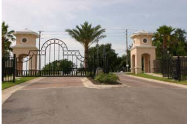
Entrance To Tower Lake Through Electronic Gates
